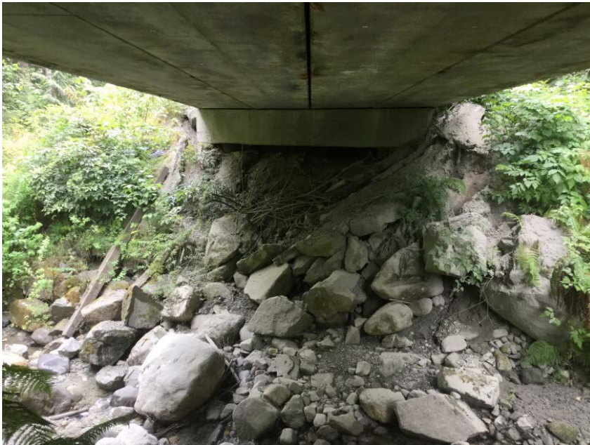
Right Bank Abutment when facing downstream
