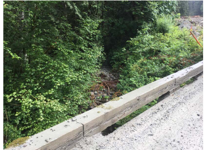
Looking upstream from deck
