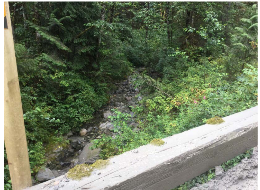
Looking downstream from deck
