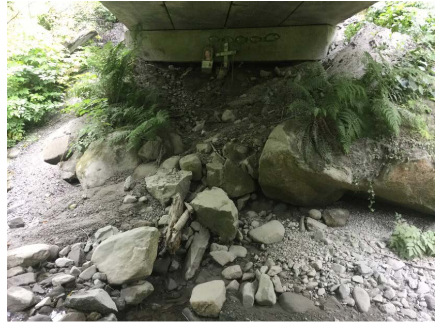
Left Bank Abutment when facing downstream
